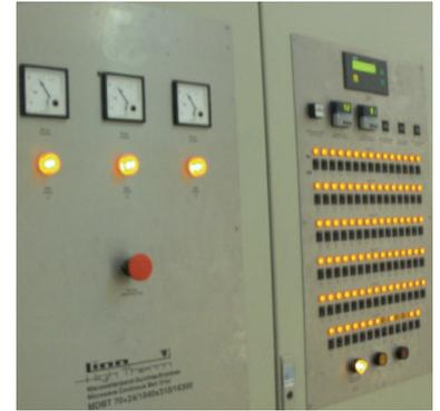
Fig. 4 Microwave continuous belt dryer MDBT 70+24/1040/210/16300 of LINN HIGH THERM in production (installed microwave power 70 kW, hot air power 24 kW, throughput approximately 2000–3000 kg/h)
